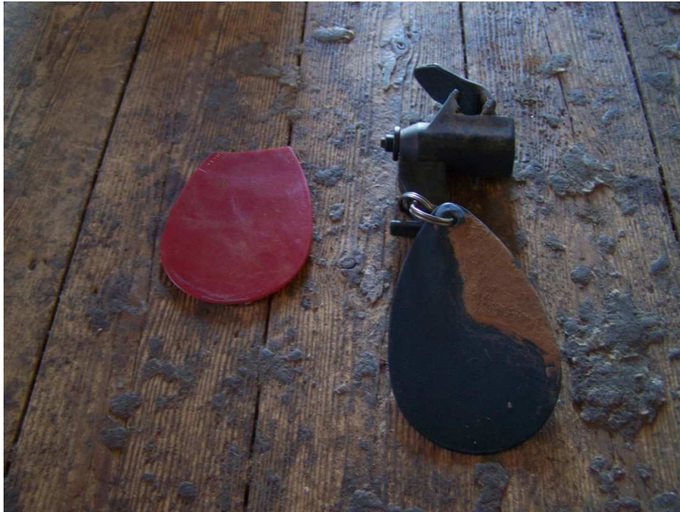
Fig. 1: The flappers that were installed in 2004. Note that the left flapper broke off in the middle and that right flapper broke at the attachment.
