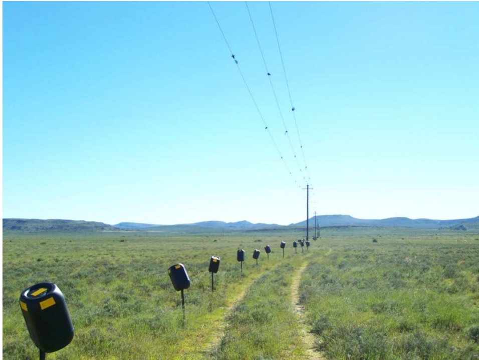
Fig. 3: The altered home-made 'barrels' with reflective tape and glow in the dark paint installed in December 2009 underneath the power lines.
